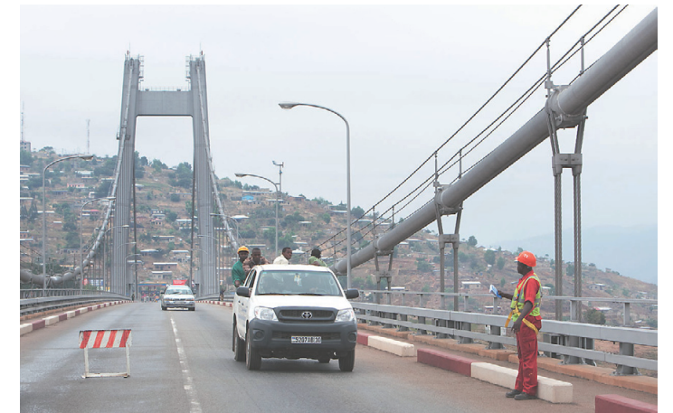
Completed in 1983 with Japanese financial and technical assistance, the Matadi Bridge spanning the Congo River is a symbol of cooperation between Japan and the DR Congo.
